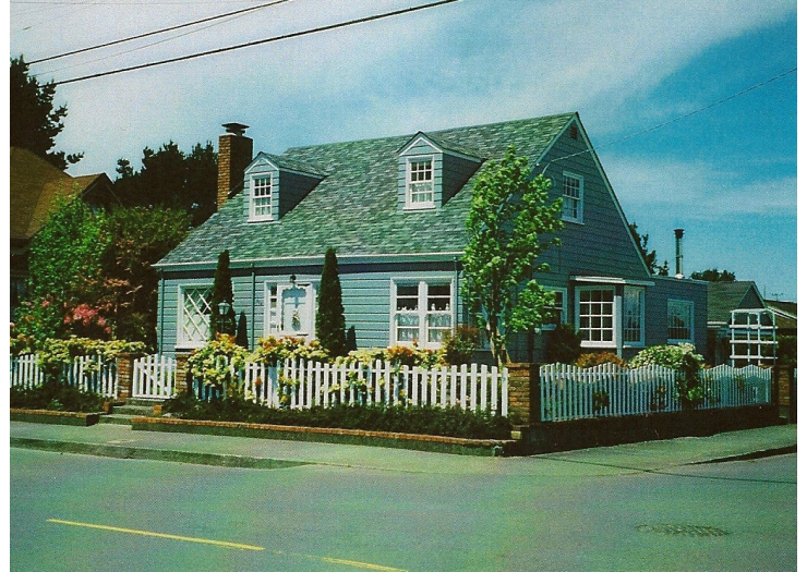
View from corner after the 1955 remodel to a Cape Cod style midcentury classic. The "L" shaped plan has been filled in, the entry is flush with the wall and centered, and a new steeper gable roof and dormers, as well as a chimney, have been added.
