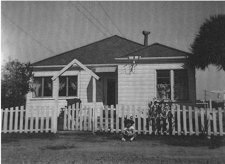
Front elevation as viewed from the street of the original 1940s cottage with its hipped roof, "L" shaped plan, recessed entry, and corner windows.
